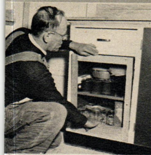
1 First, check frame for fit in cabinet. Plane if necessary to obtain \frac{1}{8} -in. clearance at each edge.
