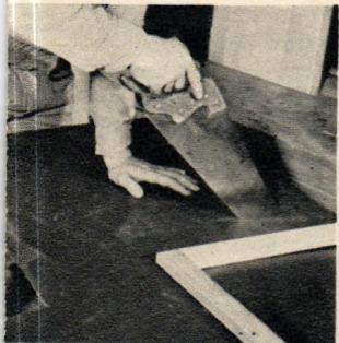
3 Use a fine-tooth crosscut saw. Cut carefully so that the line is barely visible on the cutout portion.
