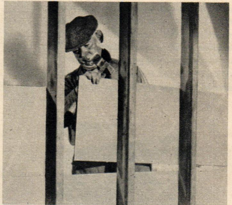
Insulating ROCKLATH plaster base fits snugly in installation, 16x48-inch panels bring joints squarely to center of studs spaced 16 inches apart. Aluminum foil vapor barrier faces outer wall, requires air space of only \frac{1}{4} -inch when used with solid masonry.
