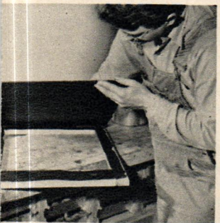
5 Spread adhesive over the frame with a spatula, then press hardboard in position for nailing.
