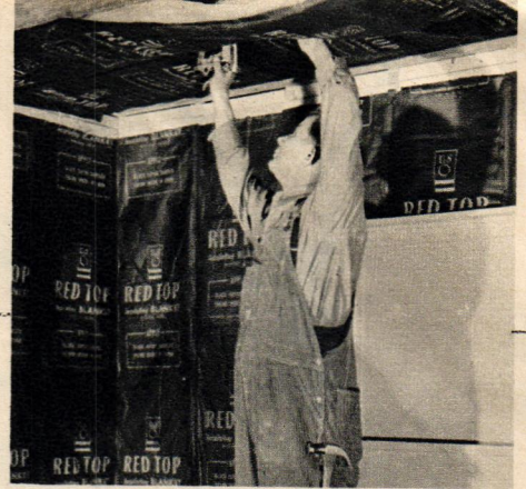
Blanket batt of RED TOP insulating wool is stapled through nailing flange into face of stud. Black vapor barrier side of blanket always faces inside. Batts come in 15x96, 15x48 and 15x24-inch sizes, in medium and thick (2 to 3-inch) thicknesses.
