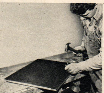
6 Drive \frac{3}{4} -in. brads through panel about 4 to 6 in. apart. Sink the heads below surface with nail set.
