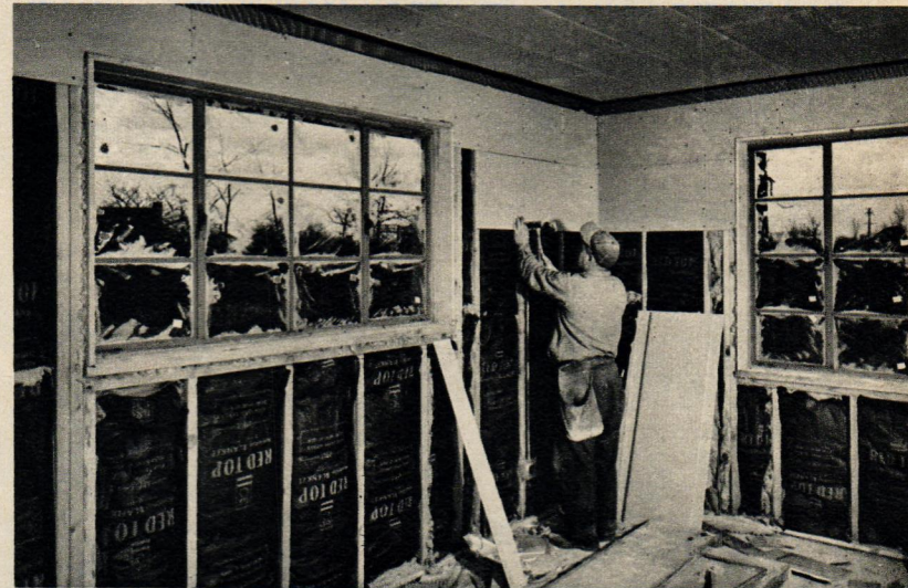
RED TOP Insulating Wool and ROCKLATH Plaster Base are in this wall
