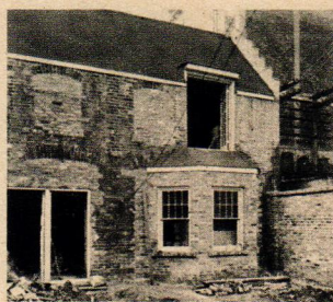
Before. Remodeling started, showing addition of new bay window to front wall.
