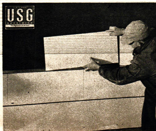
This siding stays white—never needs paint. Each course of GLATEX Asbestos Cement Shingles is attached firmly to SHADOW-LOCK channels that form pleasing shadow line.
