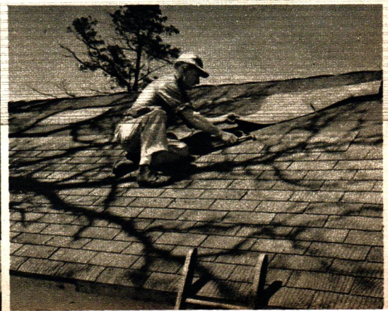
Given new lease on life, roof is recovered with USG Thick Butt asphalt shingles, laid 4 inches to the weather. Shingles go on directly over old roofing.
