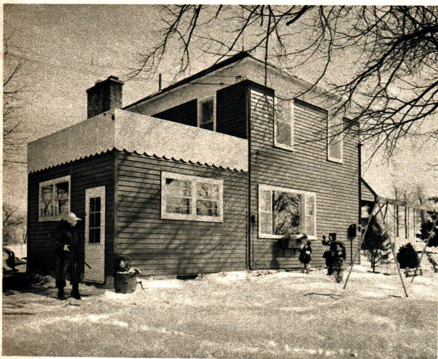
Now. New addition at rear of house is porch-workshop with convenient closet (see floor plan below). New rear grade entry makes it possible to go to basement or up into porch and rest of house with minimum of steps. New rear entrance is handy to driveway and rear lawn. Note new picture window in kitchen dining area.
