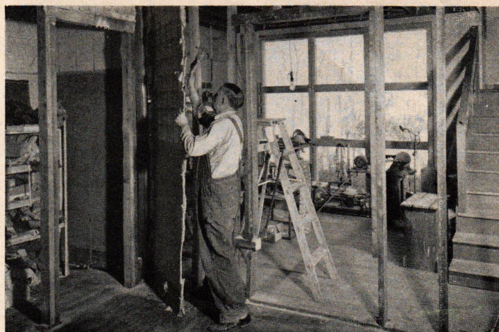
Patsy's grandfather, Neil Mackenzie, took a hand in much of the remodeling. Here, with the addition enclosed, he removes the old surface from the former back wall of the house. Next, the studs were removed to create the single large family room.
