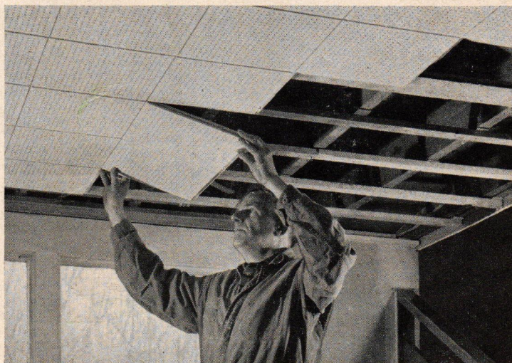
Father made sure of effective sound-conditioning by applying QUIETONE* Twin-Tile to ceiling in family room. With 1x3 furring strips in place, it was a quick job to staple up this fiber insulating tile. We found that it can be cleaned or painted, and is a "natural" for beautifying old ceilings.
