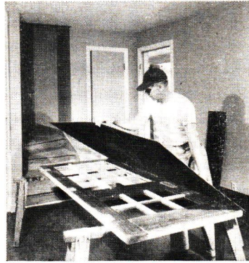
Out-of-style doors are easy to convert to flush doors. Remove glass, fit large glass openings with cross pieces for strength, face with DURON hardboard, trim edges, and paint. Doors now look new (right).
