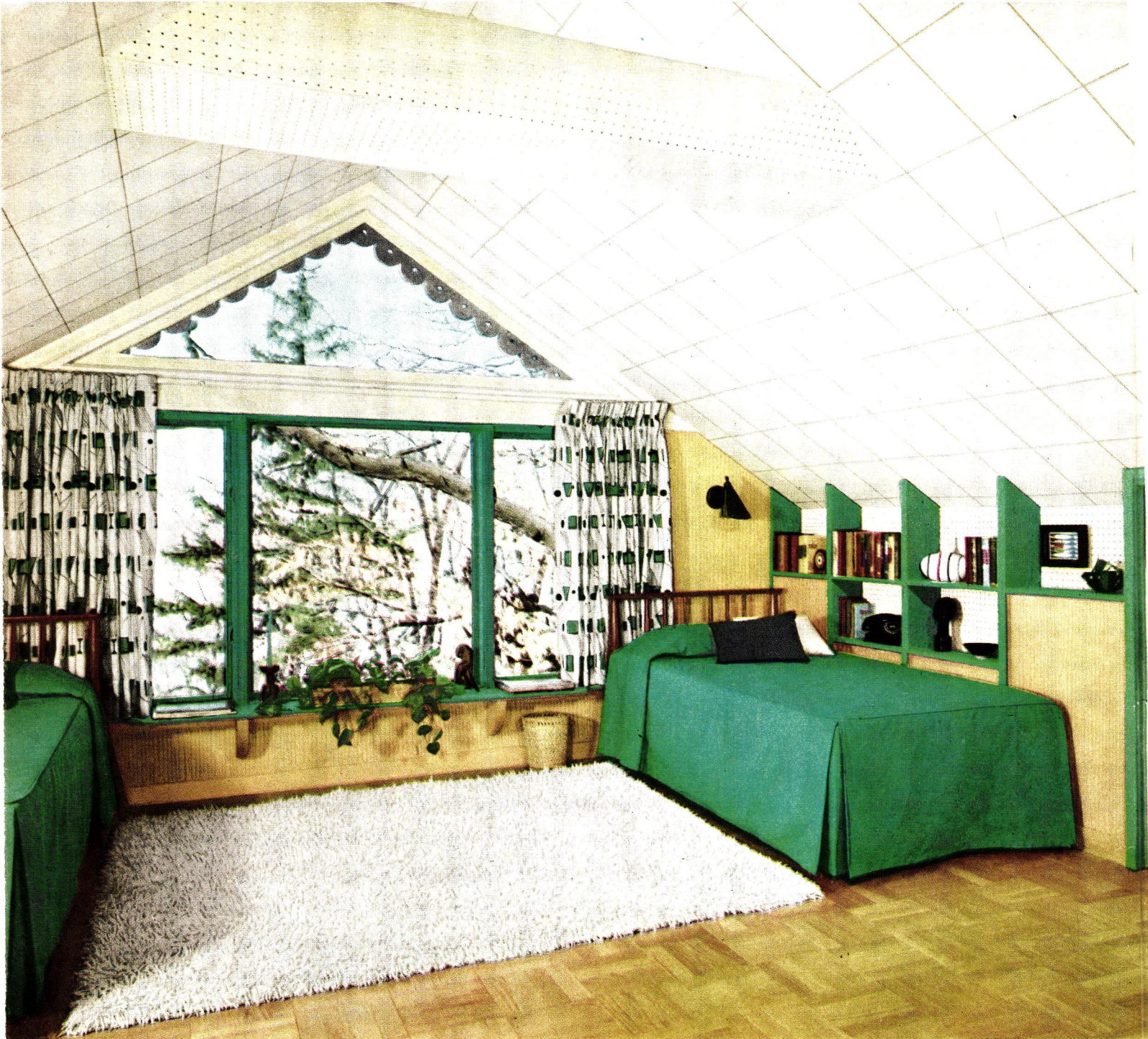
Here's a room designed for homework, play, and sleep. Knee-wall cabinet, about 4 ft. high by 8 ft. long and 14 in. deep, is constructed of \frac{3}{4} -in. plywood and 1-in. lumber with DURON Hardboard back and sliding doors. Bleached Mahogany and painted SHEETROCK gypsum wallboard are used on walls and ceiling.
