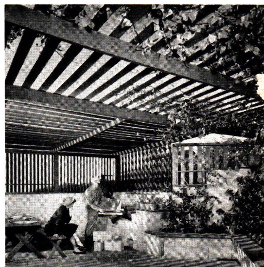
Open and shut is the case in this terrace. Concrete blocks form a retaining wall; adjustable louvers above it control flow of breeze. Slats of 1x4 on 2x6 framing plus a covering of ivy filter the sunshine and glare.
