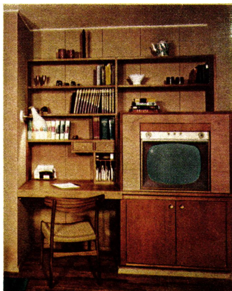
New interior wall of living room has two needed closets and a simple built-in. Because wall is cut up by jogs and doors, it has been faced with Panel SHEETROCK gypsum wallboard to improve proportions.
