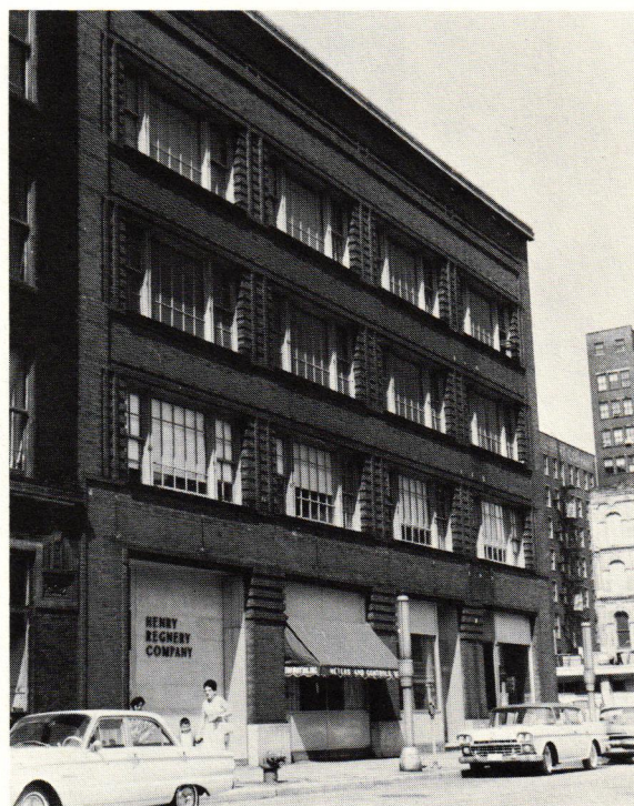
The Grommes and Ullrich building was a strictly utilitarian design in the Chicago "commercial" style. The only ornamentation was the restrained use of projecting brick courses. Photo by B. C. Greengard.
