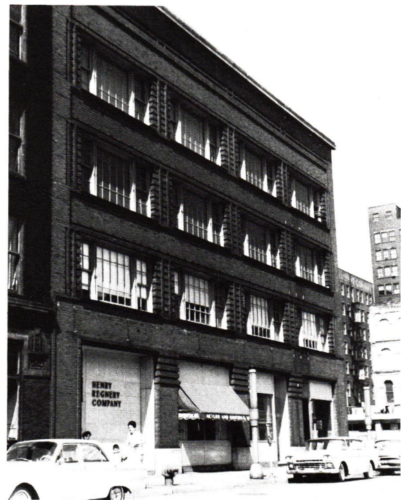
The Grommes and Ullrich building was a strictly utilitarian design in the Chicago "commercial" style. The only ornamentation was the restrained use of projecting brick courses. Photo by B. C. Greengard.
