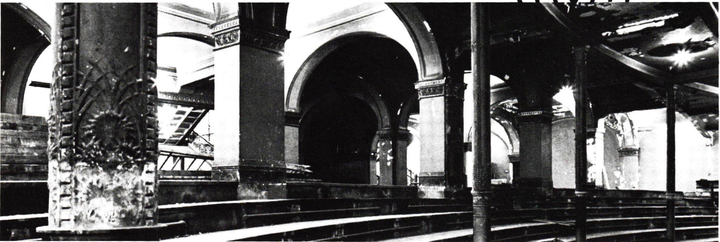
The theater was virtually abandoned for over twenty years during which no maintenance was done. Superficially it was in deplorable condition before the current restoration. Photo from the Auditorium Theater Council.
