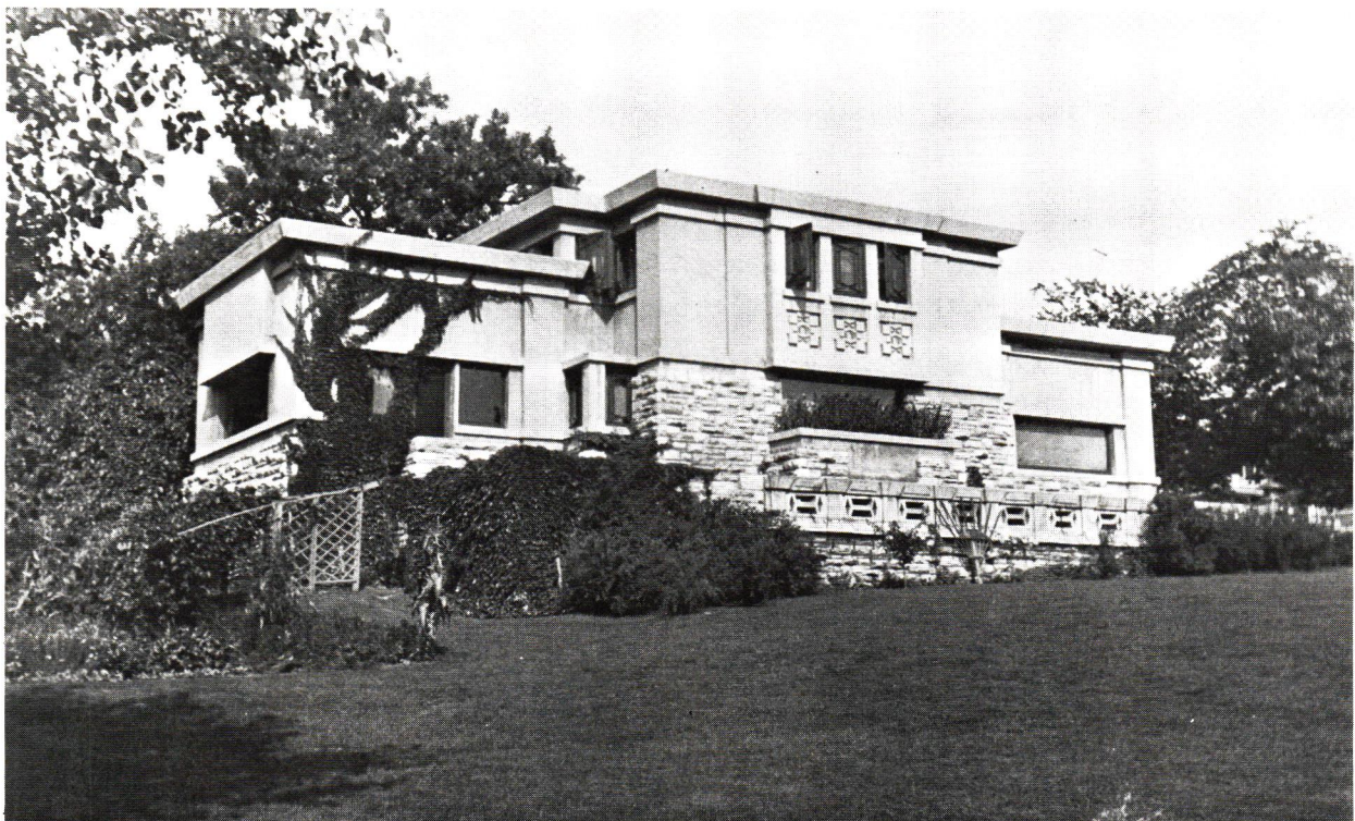
The east elevation of the James Blythe house as it appeared shortly after completion. A few minor alterations have since occurred but it remains essentially the same and stands as an example of Walter Burley Griffin's finest work.
