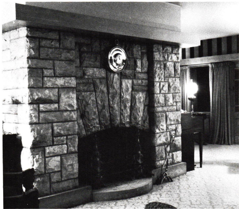
The fireplace in the Melson living room is built of similar stone to that used on the exterior, but the joints have been more deliberately dressed. The stones over the opening echo the exterior design.
