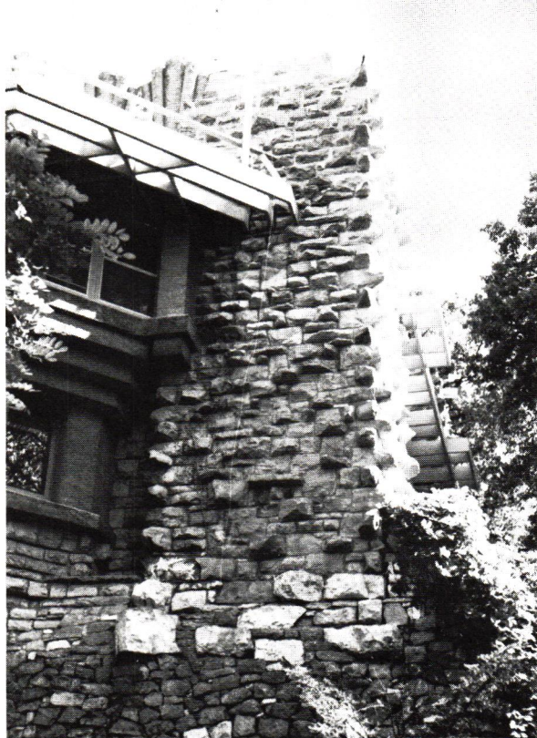
The north face of the Melson house is an extension of the natural stone cliff rising from the floor of the Glen below.
