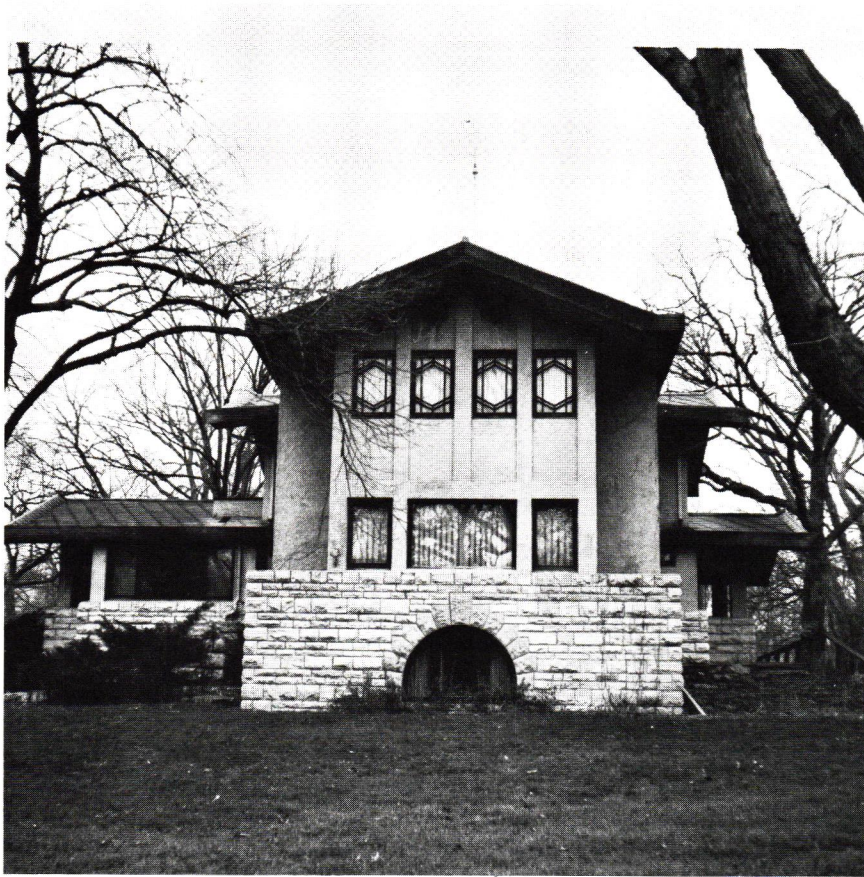
The east elevation of the Page house as it is seen from the creek. The wide central window was originally two windows identical to those on the sides.
