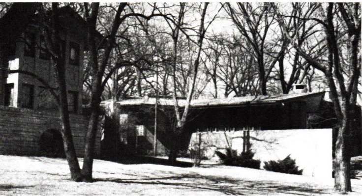
The McNider house seen from the southeast showing its relationship to the Page house.
