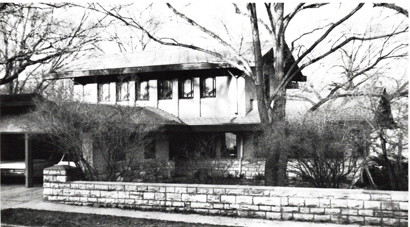
The Page house as seen from the street or west side. The garage was added after the house was completed. It was not part of Griffin's original design.
