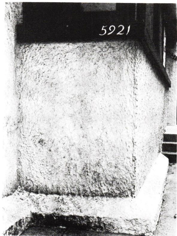
This is a detail of the base at the exterior of the house on 5921 North Magnolia. Griffin and other Prairie Architects often used a flared base such as this, but it is seldom seen covered with stucco. Generally it is of exposed wood.
