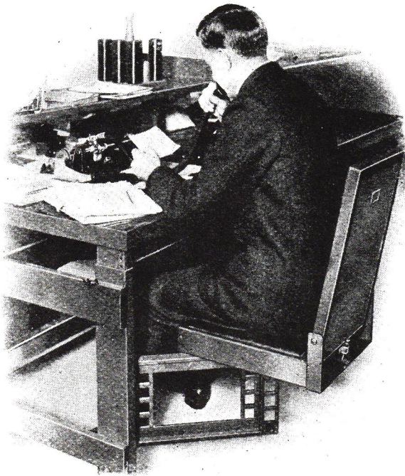
The steel desks and chairs for the Larkin building were designed as a unit. The desk tops were of magnesite.
