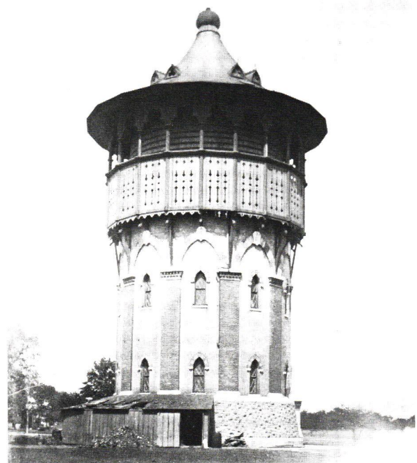
The Riverside water tower, designed by Jenney about 1871, is still standing although the roof has been replaced. It was designed basically as a "Swiss Gothic" building with "a high sloping cut stone base".
