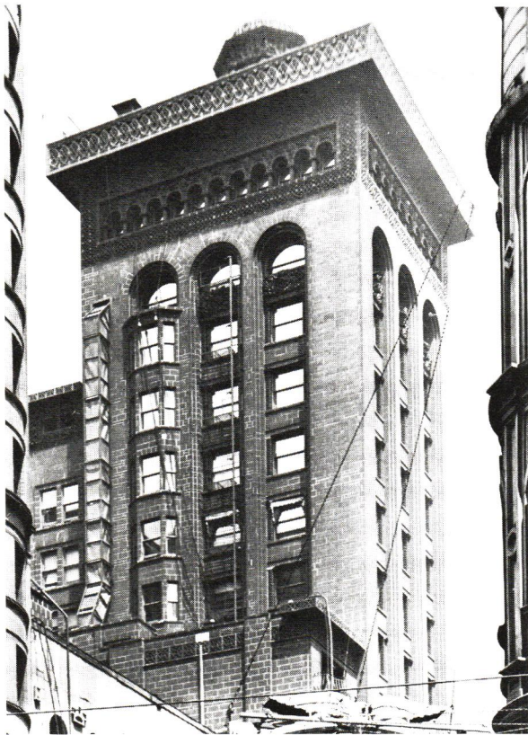
The eaves of the Schiller Building were removed, but the decorative embellishments on the facade were left intact. The ornamental panels between floor levels can also be seen. Photo by Richard Nickel.
