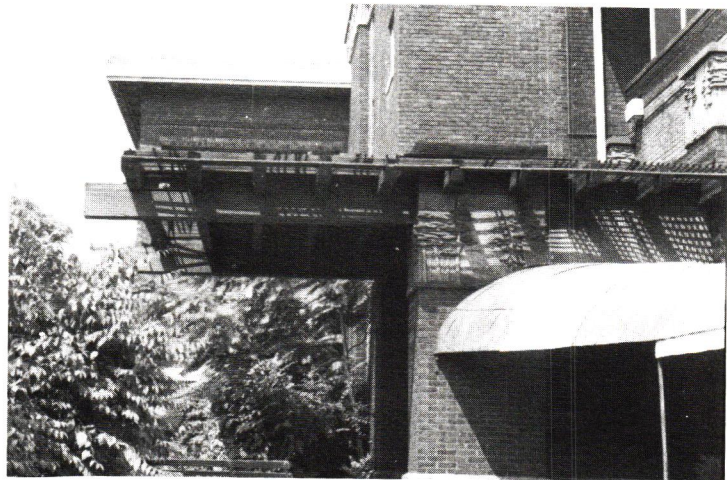
The awning of cantilevered beams suggests that Roberts may have known the work of some West Coast architects.
