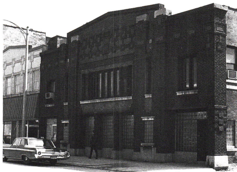
Different shades of brick create a geometric pattern ornamenting this Playhouse Theater of 1913.
