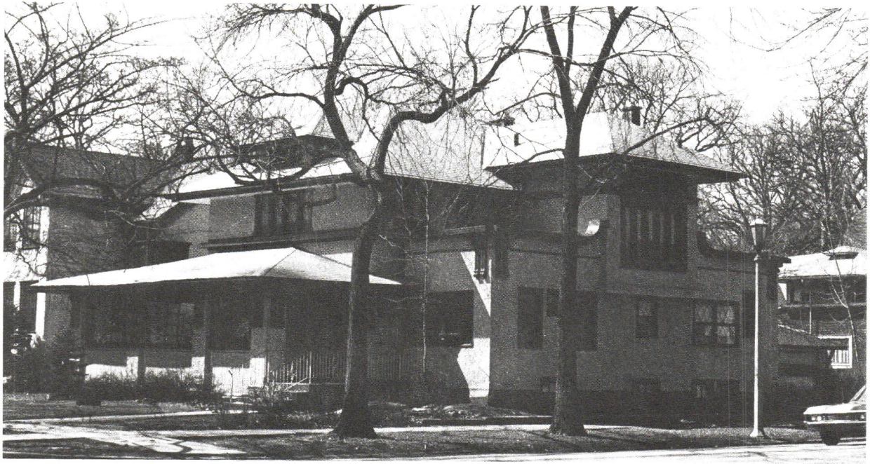
The north facade of the Melville house presents an unusual special arrangement.
