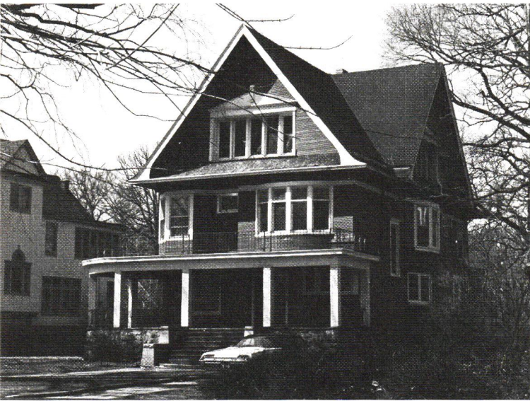
The Joseph Dunlop residence. By 1896, Roberts' Queen Anne houses were attaining a greater rectangularity than his earlier ones.
