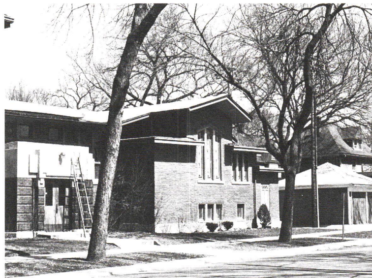
Flat side roofs contrast with the slightly sloping central roof of Trinity Lutheran Chapel, 1909.
