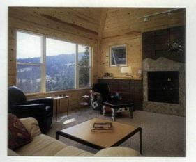
Dengler's palette of interior materials includes walls of tongue-and-groove pine, galvanized metal, and concrete block; sealed concrete floors; and sandstone counters and fireplace surrounds.
