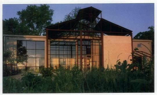
A wall of glass replaces the original overhead garage doors. Levine and Moore added the porch, supported by a 25-foot-high grid of purposely rusted steel columns that are the building's sole exterior ornamentation. Renovation costs were \$59 a foot.
