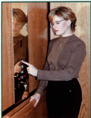
Illuminated push button car and landing control stations.
