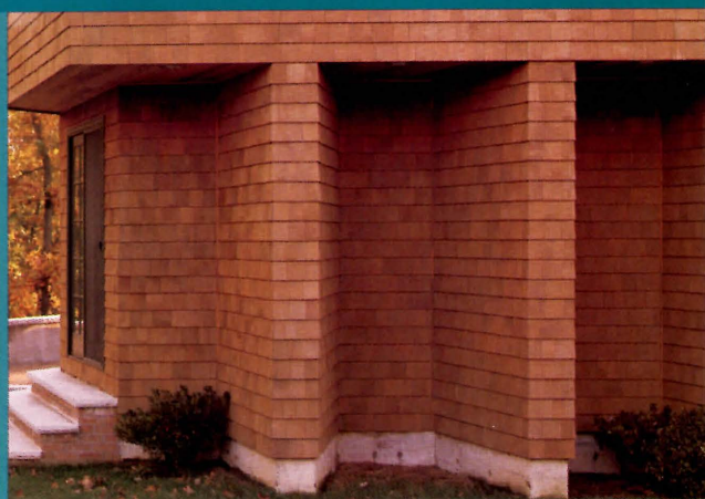
Cedar Valley Products: 4-course (5.3" exposure) shingle panels with matching prefabricated flush corners and custom angled corner returns and window insets.
