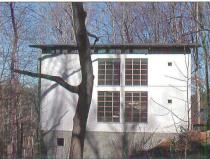
▲star glazing Harmon specs Polygal polycarbonate glazing because it's less expensive than glass, yet stronger and more lightweight. Suitable for indoor and outdoor applications, the heatreflecting, corrugated sheets can be tailored into almost any configuration. Vincent Petrarca, an intern architect at Harmon's firm, used Polygal flat transparent panes for the windows in his own home, shown. Polygal Plastics Industries, 800.537.0095; www.polygalusa.com.
