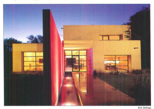
For the glazing on this home, Jon Anderson speced Kawneer's 451 aluminum system in anodized black, which contains 1-inch insulated glass and an operable section that blends with the frame.
