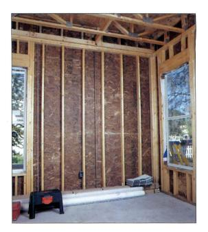
Treated with a liquid copper–based chemical, Potlatch's OXTerminator specialty OSB provides protection against termites, fungal rot, and surface mold growth.
