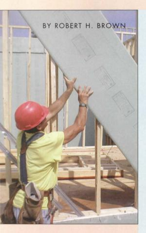
A construction worker pushes a gypsum board area separation wall liner panel into position at Chalfont Greene, a townhome development north of Philadelphia.
