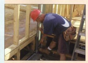
A framer at Chalfont Greene fastens a breakaway clip to the steel framing of a gypsum board area separation wall panel (top photo) while a co-worker secures horizontal track that will hold in place two layers of gypsum liner panel.
