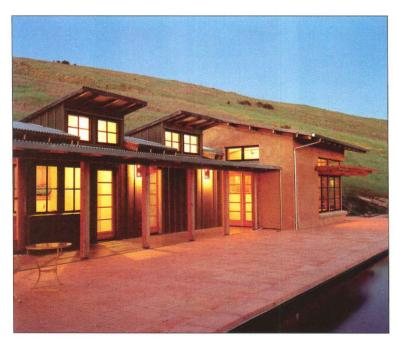
The 18-inch-thick main walls of this vacation compound in Sonoma County are made from rammed earth. Smaller buildings house the bedrooms and baths. A 3-inch-thick bowling lane tops the kitchen island; old glass bottles form the bathroom counter.
