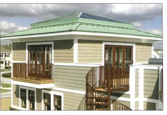
Structural insulated panels, a roof with low-E coating, and electronically tintable glass windows and skylights help to create a durable, energy-efficient building envelope at the Not So Big Showhouse.
