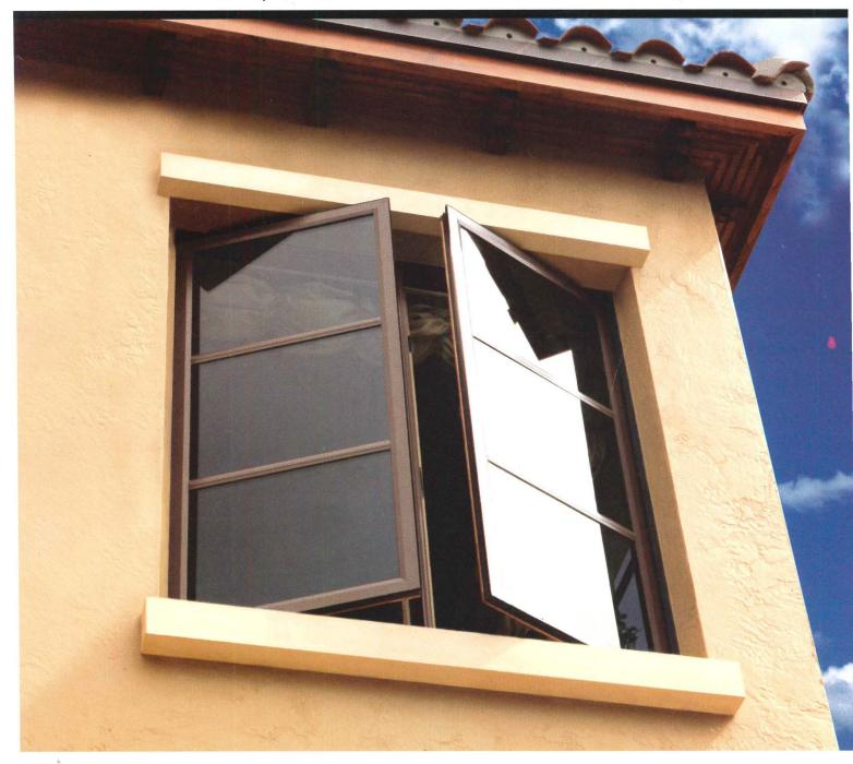
Shown above: Anodized dark bronze aluminum exterior Weather Shield® casement windows. This is one of seven anodized colors offered by Weather Shield. Each provides lasting beauty that resists chipping or peeling, even under intense exposure to the sun. For complete sizing and ordering information, call 1-800-477-6808 or visit weathershield.com/RA
