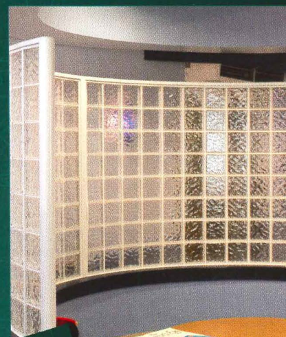
Round caps finished off the ends of this radius wall. Aluminum mullins were used to connect the three radius walls together, while a flat cap mounted the units to the top of the curved wall.
