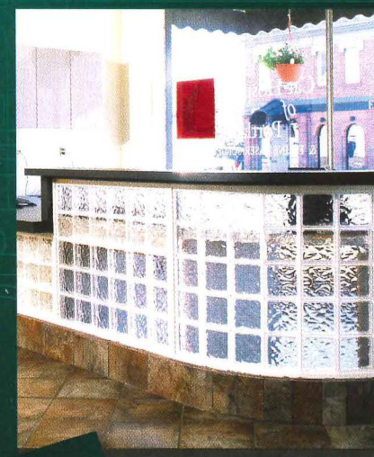
Aluminum mullins were used to connect these flat panels and radius walls together. A flat cap and mounting channel were used to mount the units to the base and the walls. Flat caps were also used to connect the desktop to the top of the partition.
