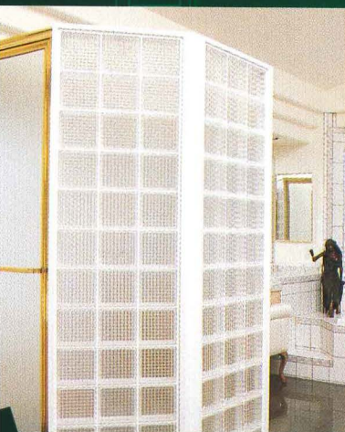
45-degree corner caps were used to connect Hy-Lite panels to form this neo-angle shower. Flat caps were used to finish off the top and sides of the doorway, while a flat cap and mounting channel were used to attach the panels to the curb and wall.
