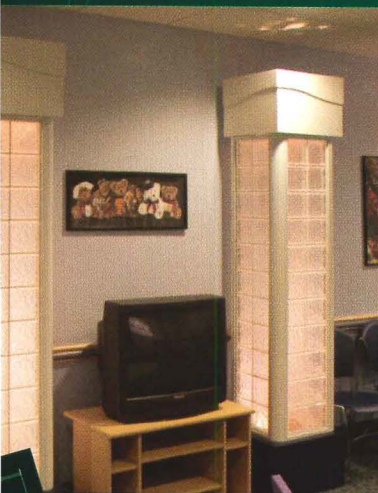
90-degree corner caps were used to connect four acrylic block panels together to form decorative, lit towers. The panels were mounted to the base and top piece with flat caps.
