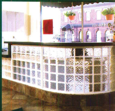
Aluminum mull were used to connect these flat panels and radius walls together. A flat cap and mounting channel were used to mount the units to the base and the walls. Flat caps were also used to connect the desktop to the top of the panels.
