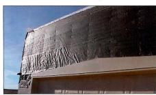
The wrinkles in the Secondary Weatherproof Membrane will cause thick and thin spots in the basecoat. These will have different expansion and contraction characteristics side by side and will stress the stucco assembly.
