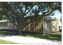
Photos (above and top): Courtesy Studio 804 Studio 804 built its first prefabricated house in 2004. Modular 1 (top) consists of five modules, each dedicated to a different function. Modular 2 (above) incorporates maple flooring from an old gymnasium and leftover channel glass from a nearby museum expansion.
