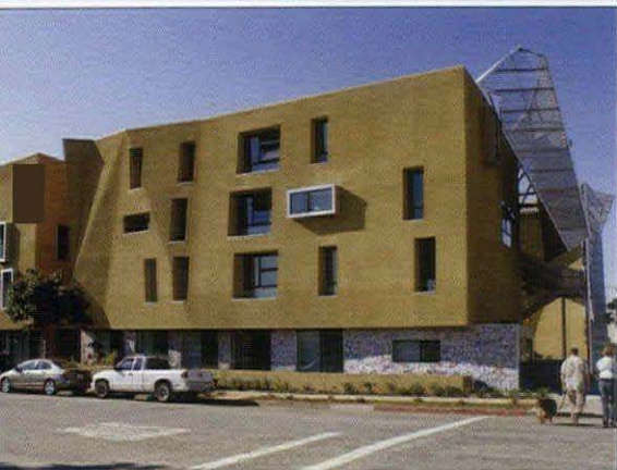
Protruding and receding windows add visual depth on the east side. The building is chock-full of environmentally friendly materials, including accent cladding of custom-pressed blocks made from recycled cans (right and opposite).
