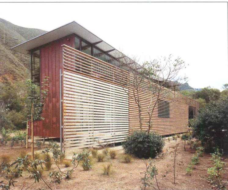
Stilts reduce the Jackson Family Retreat's impact on the land and protect it from flooding if a nearby creek overflows. Cedar slats screen the front façade from the road, while the rear of the house opens to nature.
