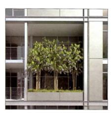
Shalom Baranes Associates covered the 22 West condo building in a durable zinc cladding that has a naturally warm patina and inherent green properties. The firm specified a module installation that produces very little waste.
