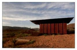
Practical, impervious, and low-tech, the cargocontainer guest cabins are at home on the harsh Texas range. The five containers—three bedrooms, a kitchen, and storage space—are linked by a deck of steel bar grating with built-in bench and barbecue.
