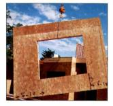
Panelized construction systems, such as the structural insulated panels from Premier Building Systems (above) and this wall from Weyerhaeuser's iLevel business (left), allow architects and builders to cut construction time, lower labor costs, and reduce waste. Pricing compared with on-site stick framing, however, depends on many factors.
