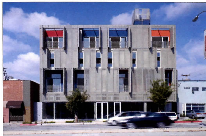
Residents can change the building's exterior appearance by opening or closing their units' perforated metal screens.
