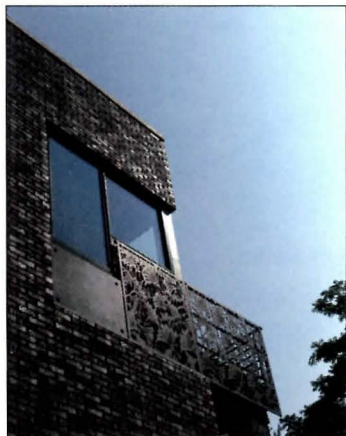
The building's exterior is highlighted by glazed metallic brick and Cor-Ten steel panels with ginkgo leaf cutouts adapted from a traditional Japanese paper carving.
