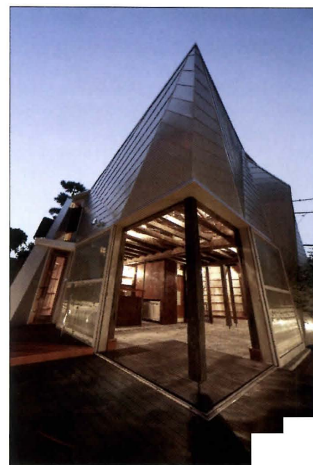
Two 100-year-old timber-frames, relocated and combined, form the structural system of a new house (left). Galvanized steel-faced sandwich panels wrap the building in a modern skin (top), and corner sliding doors open onto a private terrace (above).
