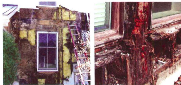
Water damaged walls.
