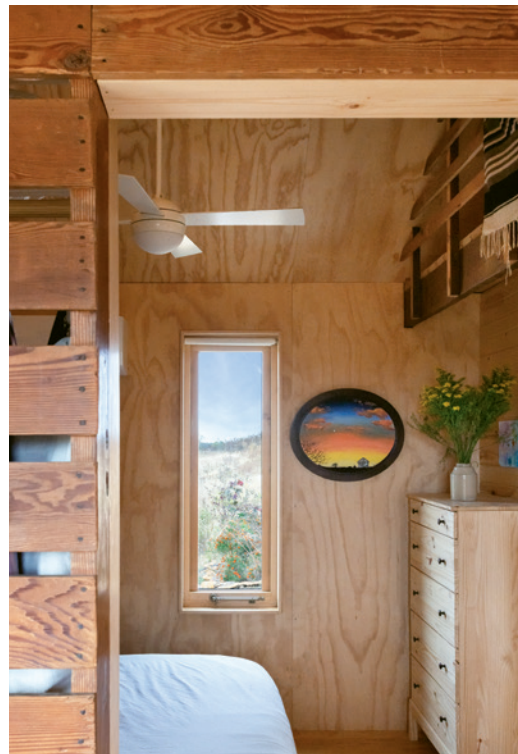
Windows were slipped between existing studs to preserve both the building's aesthetic integrity and its strength in a tornado-prone region.
