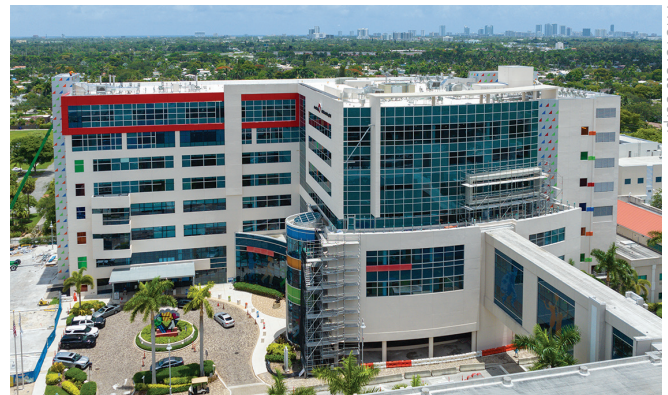
The existing building's stucco had been installed without properly leveling the building. Once the old stucco was removed, the existing building and new addition were married together seamlessly.
