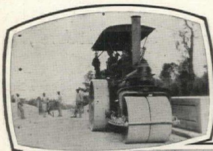
F. A. P. 32—10 miles. Penetration Slag Macadam in Nassau County between Callahan and Jacksonville, Fla.
