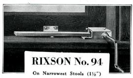
this Operator opens Outswinging Casements in 3½. Turns of the Handle, does not disturb Fly Screens and Locks at any point Positively and Automatically. Write for details, or see Sweet's Catalog
