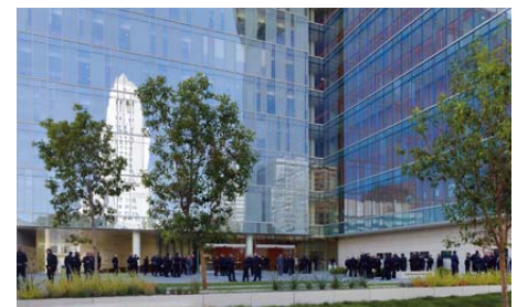
Photo: Tim Griffith
