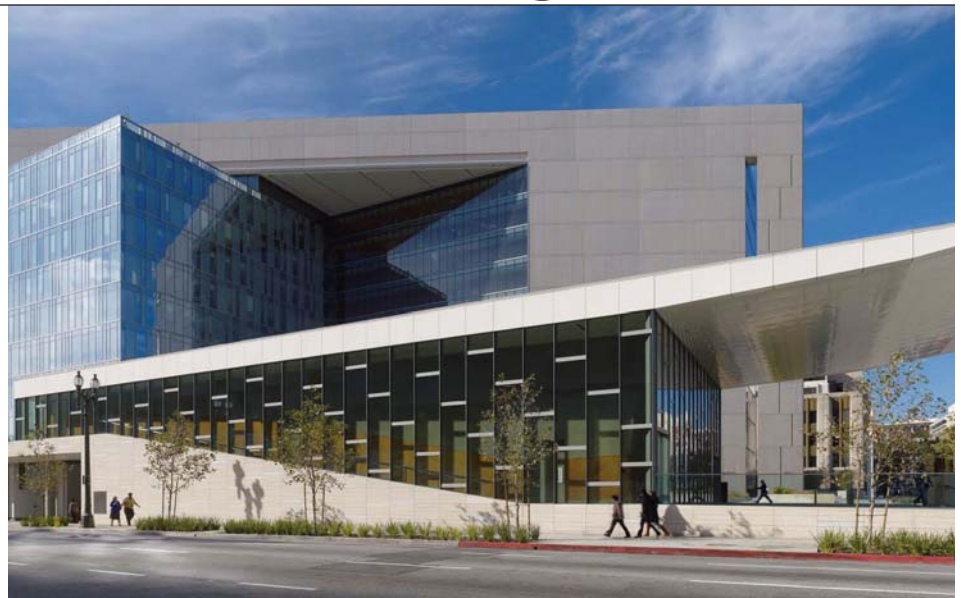
Photo: Tim Griffith
