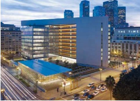
Photo: Tim Griffith
