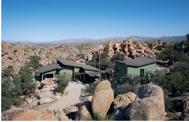
Weekend Cabin in Yucca Valley by ORA Architecture & Design. Photo: Eric Staudenmaier
