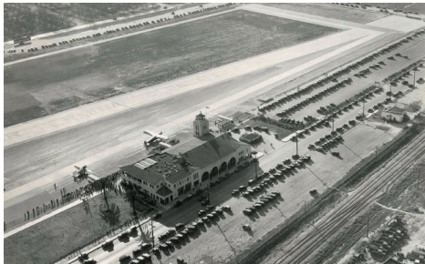
Aerial view of Grand Central Air Terminal in Glendale, February 28, 1932.
