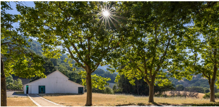
The old barn on the O'Neill property was originally built when the property was used as a cattle ranch outpost. Photo: Saxon Holt/PhotoBotanic
