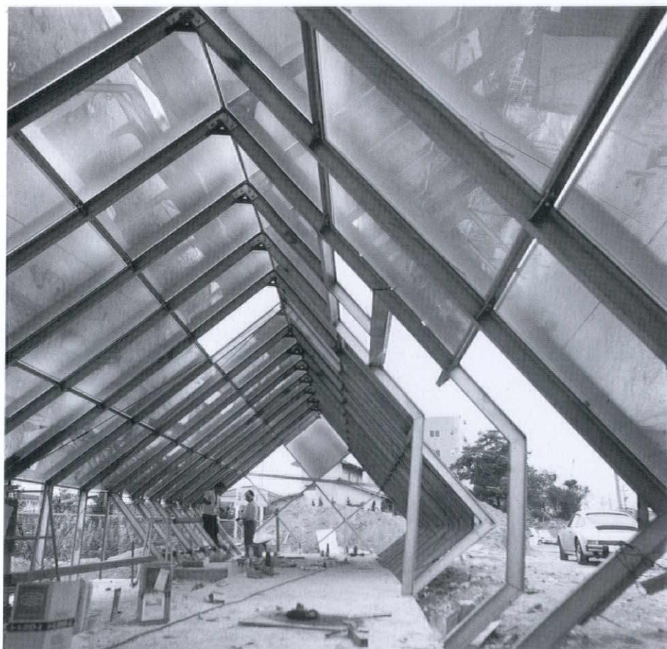
Cushioning silicon structure glazing.
