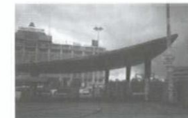
F | OMA バス停 | 1987 Bus Station 1987 Stationsplein 1 Rotterdam
