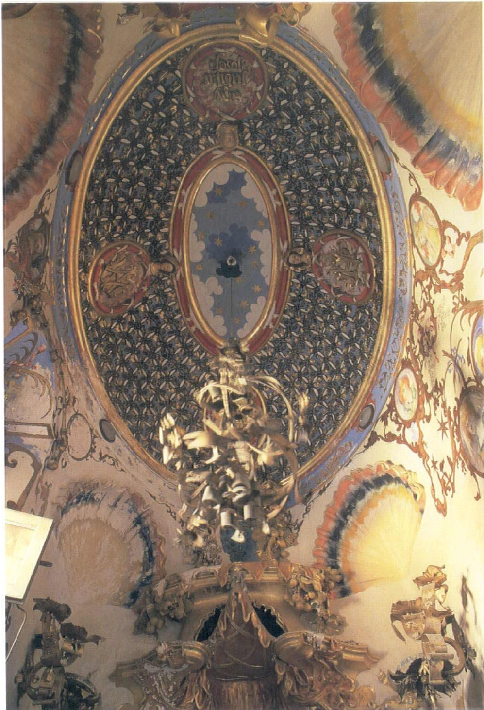
祈禱室天井見上げ
