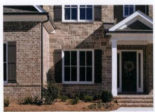
THE SKINNY ON THIN Manufactured masonry veneers offer a host of styles suitable for both interior and exterior applications.
