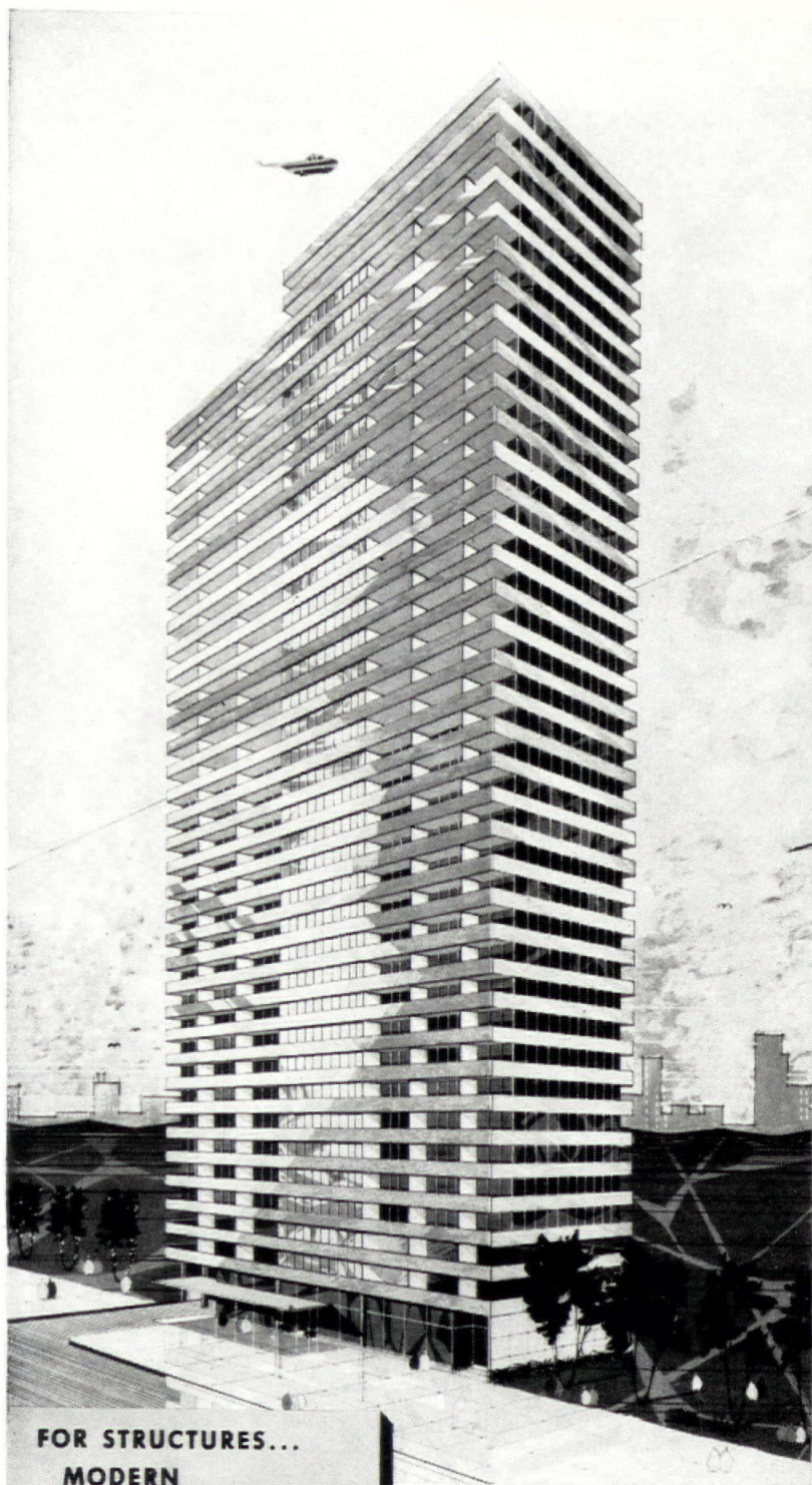
Four concrete shear walls extending across the width of the building provide necessary resistance to wind forces.
