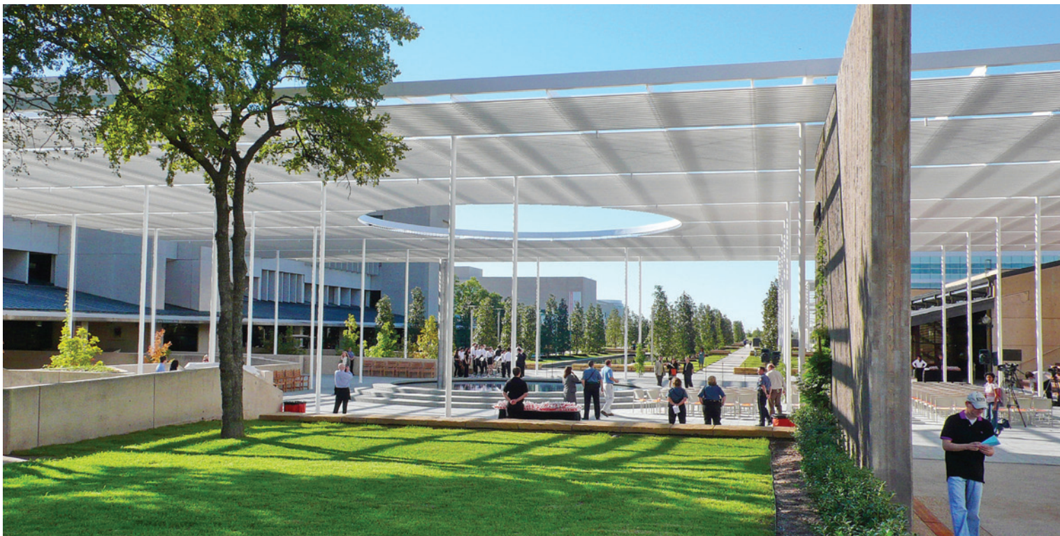
top and below The trellis, designed by Werner Sobek, is made from painted steel columns and beams that support fiberglass and plastic tubes. New construction will add 280,000 square feet to the campus by later this year.
