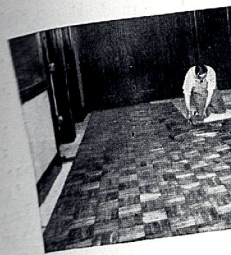
Laying *CELLized oak floor blocks in EVERBOND over a wood subfloor in a Chicago office building
