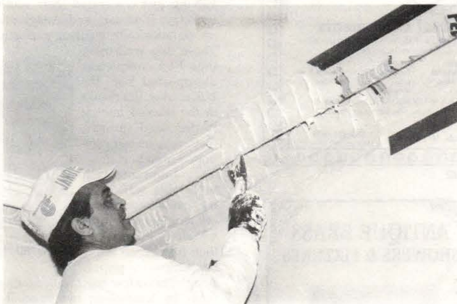
Peel-Away I is applied like joint compound to a depth of about 1/4 in. on the surface to be stripped. A test patch establishes optimum thickness and soak time.
