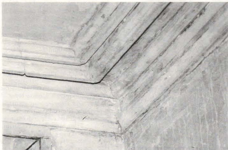
After soaking for 24 hr., the blanket is stripped off, peeling the paint with it. Disposal of paint-laden blanket should comply with regulations for lead materials.
